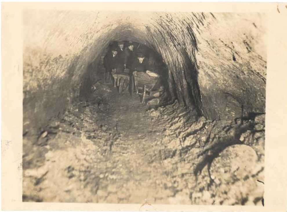
Excavating the Western Passage
